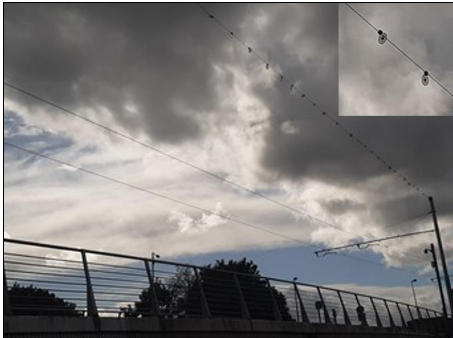
Figure 8-5 Bird deflector/ flight diverters on the Anne Devlin Luas Bridge, Dublin.
