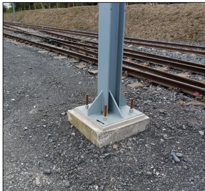
Figure 8-4 Existing catenary pole foundation at the MSDC (pen for scale)
